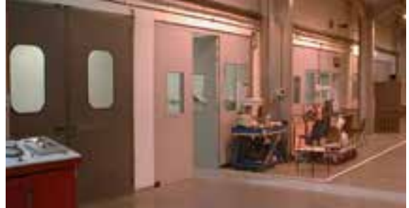
Purpose built pressure test bays
