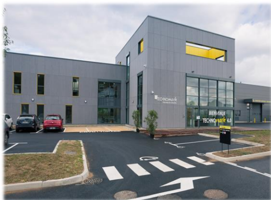
TECHNOMARK (France) HEAD OFFICE & MANUFACTURING
